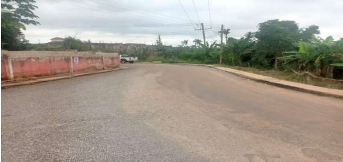
Bitumen surfacing of Greenland Street in Agona Swedru
