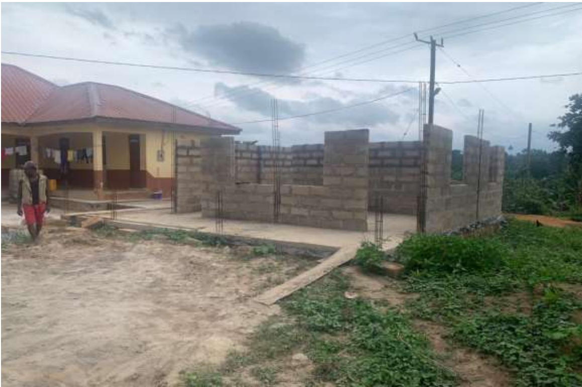
Construction of Adolescent Weighing Centre in Ahamadonko
