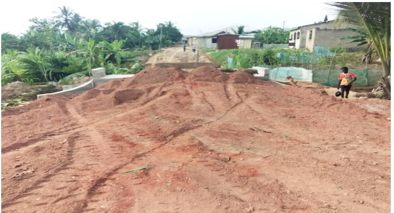
Culvert construction at Wawase
