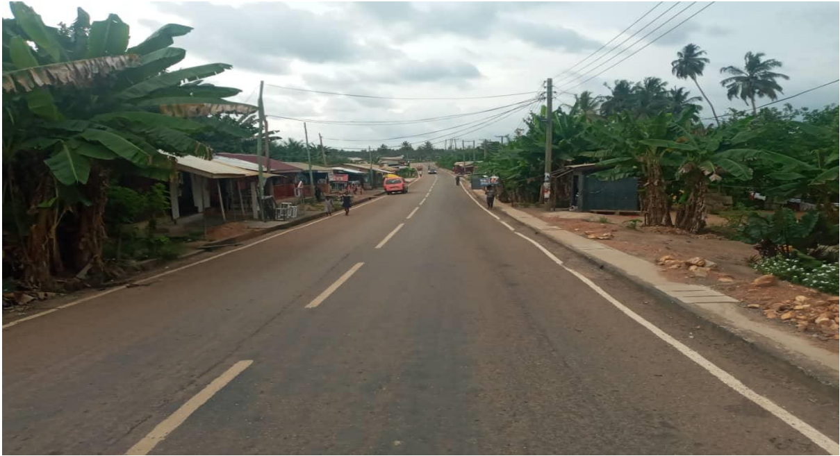
Bitumen surfacing on Esukontsen street (0.73km)
