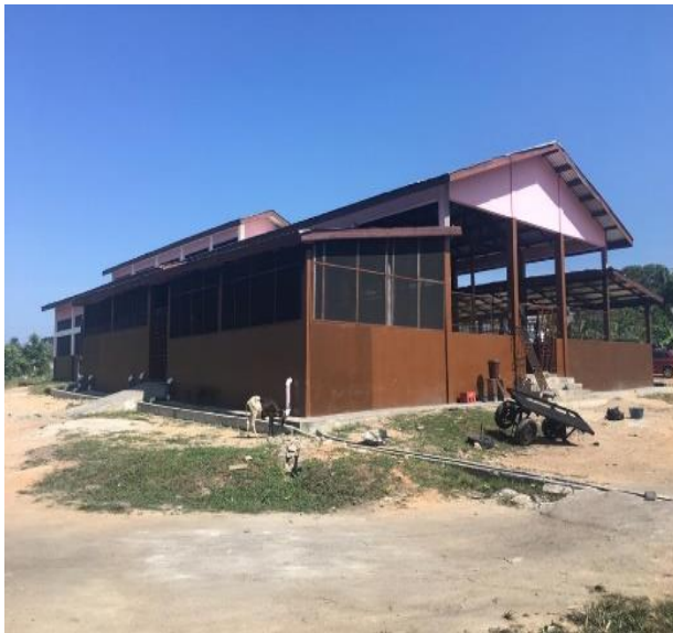
Completion of Abattoir at Agona Swedru.
